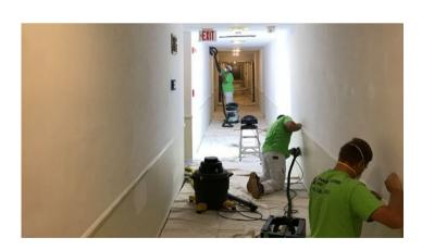
Note: Ask that the floor be protected with brown construction paper during construction. Cove base should be protected as well. Do not use the red paper as it can bleed into the floor and stain it.
